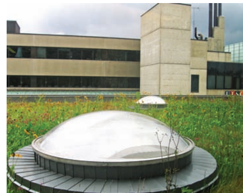
Figure 3.20 A “green” roof includes soil and plants that absorb water as well as heat in the summer to keep the building cooler.
